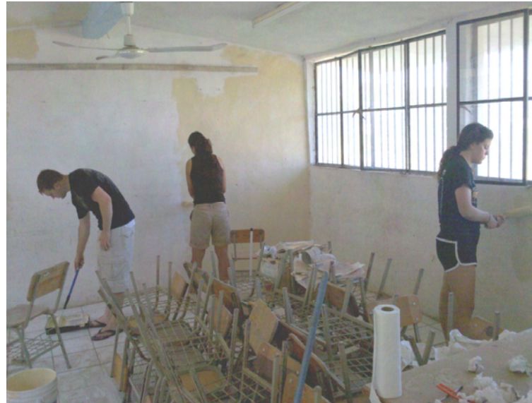
Ft. Hays University on the job
